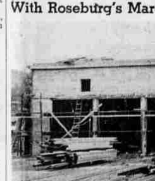
CONCRETE REPLACES WOOD —Ford Lumber Company is replacing with concrete the wood structure formerly housing the huge dry kilns at its plant on East Second Avenue South. It will be re-assuring and no doubt surprising to many to learn that an attempt even is made in these days of haste to dry lumber.
