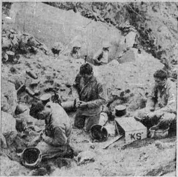
Amid scattered shell cases in front of a demolished concrete bunker, these Marines pause for prayer and communion before heading back into battle for Iwo Jima.
