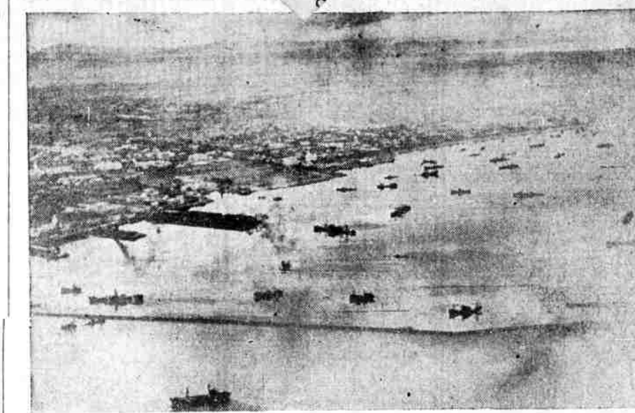
MANILA HARBOR GRAVEYARD FOR JAP SHIPPING—Dramatic proof of effectiveness of navy carrier raids on Manila bay is provided in this recent photo of the great anchorage—with more than 50 ships sunk or immobilized as result of our air raids. Waterfront installations and shoreline fuel and ammunition dumps have also felt the weight of the navy's blows. U. S. navy photo.
