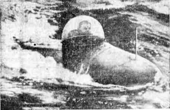
A German one-man torpedo is pictured as, like a monstrous shark, it speeds toward its objective. Actual torpedo is under water. "Driver" of the missile can be seen through transparent turret.
