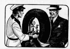
2. THEN WE VULCANIZE IT... Rubber is cemented into the hole outside; a "section repair" is built up inside replacing the broken cords. The repair is then welded into the tire under heat and pressure.
