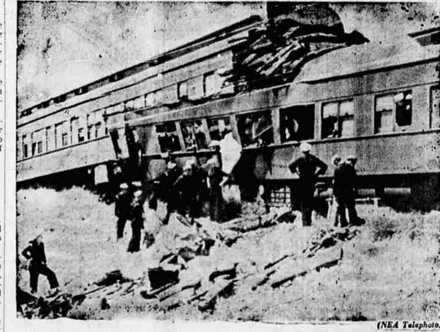
Here's how cars of a Chicago, Milwaukee, St. Paul and Pacific mainline passenger train telescoped into one another when the train sideswiped a freight train at Warden, Wash., killing nine sailors and injuring 12 others. The sheet in the passenger car window covers one of the bodies as sailors examine the wreckage.
