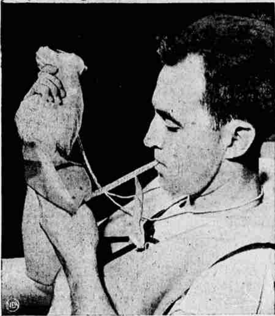
Purifying device demonstrated here by sailor converts salt water into drinking water—a boon to seamen and flyers adrift at sea. Water is put in top part of bag and squeezed through chemicals that filter it. All life rafts will carry this equipment.
