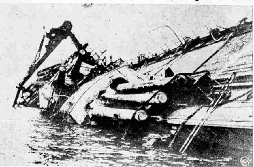
The U. S. battleship Oklahoma's days are not over yet. Blasted, with 18 other vessels, in the Jap attack on Pearl Harbor, the big battleship overturned with a large percentage of her crew aboard. Now, after months of arduous salvage work, the vessel is shown as she is righted. She is expected to sail again under her own power. Official U. S. Navy photo.
