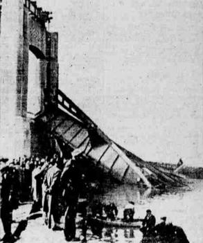
When three hune spans of the world's largest girder bridge, using constructed over the Connecticut Hiver at Hartford, Comm. collepsed and plunged 150 feet into the water. 10 workmen were killed, four missing and at least 17 others injured. Here's the shore end of the \$4,400,000
