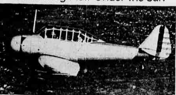
These planes represent two recent and revolutionary advances in American aviation. Above: The first stainless steel military plane ever built, an Army trainer, soars over Bristol, Pa. Use of stainless steel eliminates riveting, resulting in speedier construction. Below: flying over New York, is a molded plastic plywood plane. Besides being cheap, plywood is stronger proportionately to its weight than aluminum.
