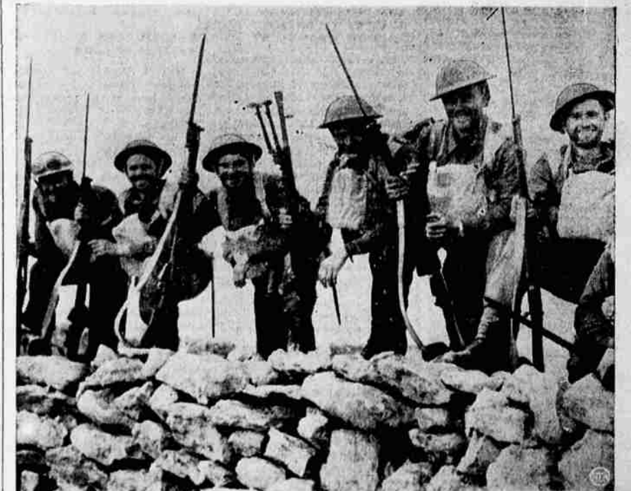
Real victory smiles are these, for a few minutes before this contingent of Aussie troops had stormed a heavily defended fort in Bardia, where the Italian general staff was directing operations. This section, alone, had the distinction of capturing three Italian generals and their staffs. "Well, we thought it was a general assault," was their humorous comment.
