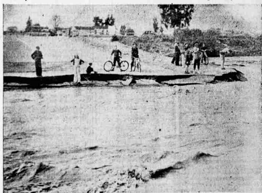
Once a main thoroughfare, Riverside drive in North Hollywood is a dead-end street as continued downpour in the Los Angeles area created a big wash that ripped out the pavement, made the road impassable.
