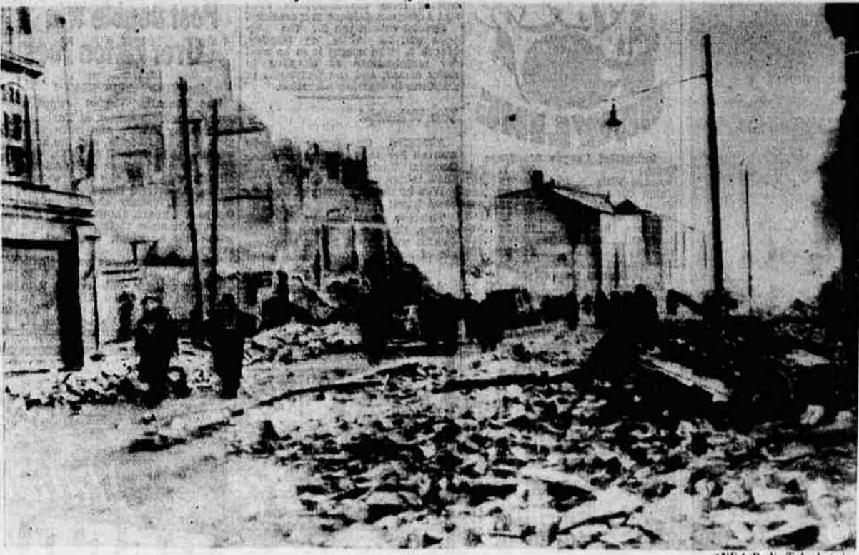
Rubble-littered streets, gutted buildings, smoking ruins of what once were homes and factories, this is Southampton, England, after England's enemy turned loose his dread Luftwaffe and its plane-a-minute technique to produce desolation and death. In this first and exclusive picture to reach the United States via radio from London homeless refugees wander disconsolately through the ruins.
