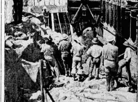
Pouring of the first concrete in what will be the second largest masonry dam in the world—on the Sacramento river near Redding, Calif.—marks the actual start of construction on Shasta dam, a part of the Central valleys water project. The eight cubic yards of concrete gushing from the bucket are the first million yards to go into dam and power plant.
