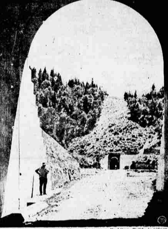
No mean part of the work at Shasta Dam near Redding, Calif., is relocation of 30 miles of Southern Pacific Railroad line—around the site of Shasta reservoir. Besides eight bridges, 12 tunnels—like the two above—must be constructed. Each of these concrete-lined bores is about a half mile long.
