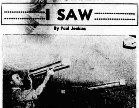
L. W. ANDERSON, Roseburg electrician, as he installed fluorescent lighting system in the Roseburg pharmacy.
