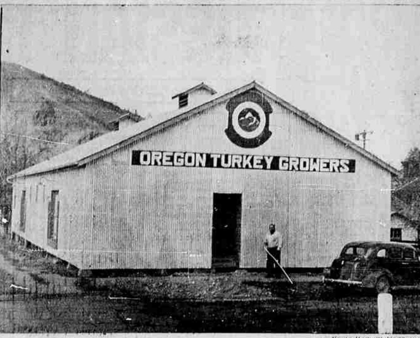
The building, dressing and shipping station, recently authorized for Roseburg by the directors of the Oregon Turkey Growers association has been completed and placed in operation. The plant, pictured above, and located at Mosher and Patton streets, affords facilities for killing and dressing with the semi-scale method. Refrigeration facilities permit pre-cooling of birds prior to packing. The method is utilized at similar plants in Canby and Eugene and is reported to provide a much better pack than was obtainable under the former dry picking system. The Roseburg station is under the management of James E. Conn, who is pictured in front of the new building.
