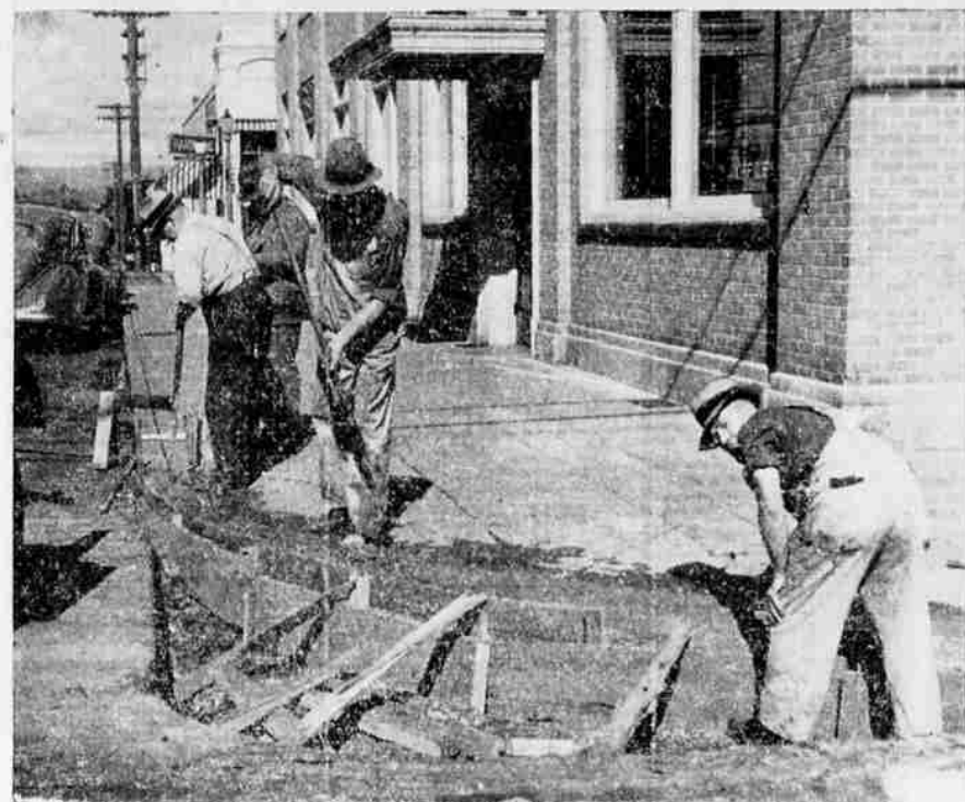
Elimination of sharp turns on congested street intersections has been proved to be a great aid in improving traffic safety in Roseburg, and sidewalk corners are being cut back as rapidly as funds are available. Shown above are members of the city street department widening the turn on the west side of Main street at its intersection with Oak street.
