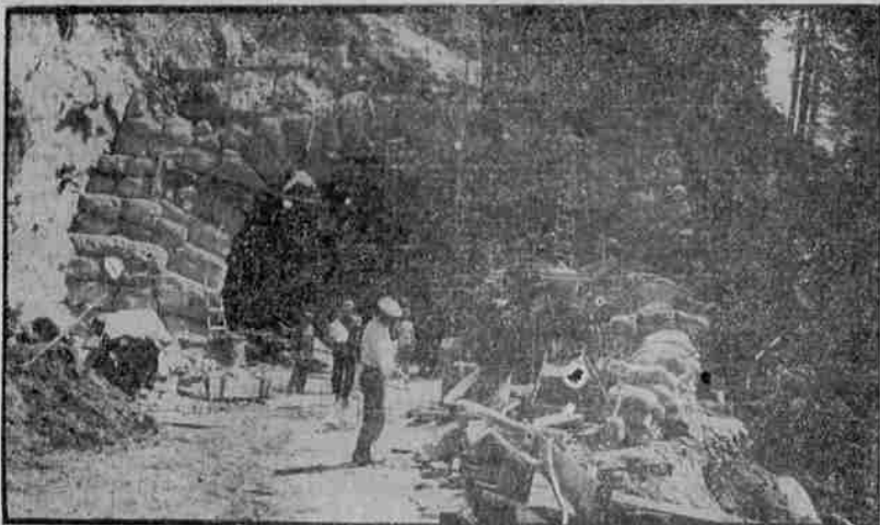
A 925-foot tunnel is being rushed to completion on the Willamette Pass highway, which will cut 50 miles from California-northern Oregon travel. Above is one of the portals.
