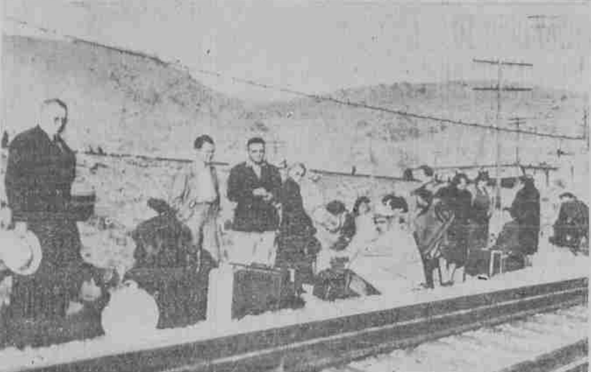
With what baggage they could save from wreckage of Southern Pacific steamlocomotive, City of San Francisco, survivors wait along railroad right-of-way near Corbin, Nev. to be picked up by rescue train. More than 20 fellow passengers were killed when train plunged off bridge over Humboldt river.
