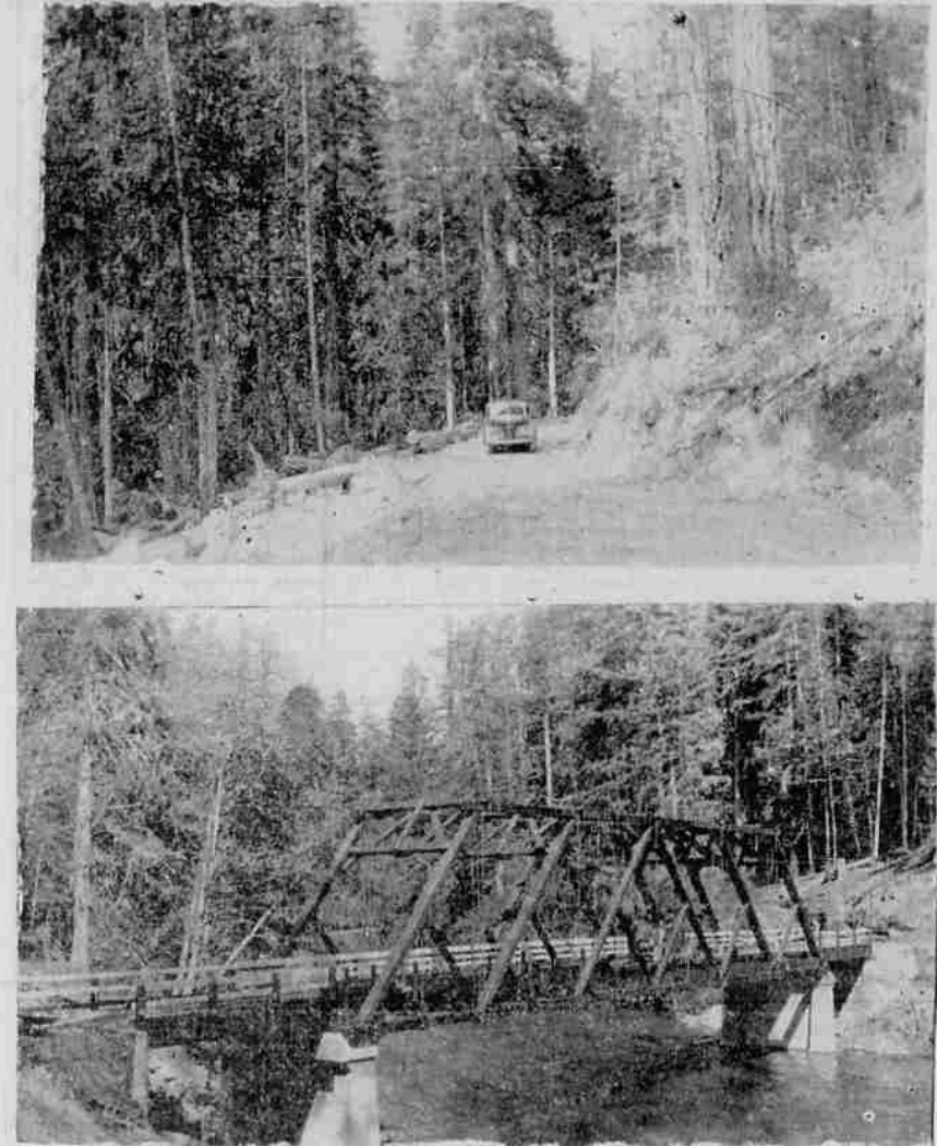
Top—Showing end of grade on North Umpqua road about 4000 feet up river from new bridge across the river. Three and one-half miles beyond here will open the road to Diamond lake. Below—New bridge finished last month by Steamboat CCC workers providing passage for equipment to complete the unfinished portion.
