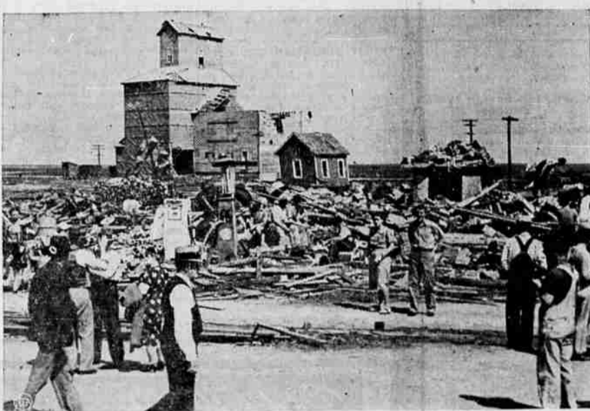
City hall, garage and grain elevator were made shambles in Capron, Okla., above, by the tornado that this week swept parts of eight southern states, killing 49 persons and injuring at least 350 others. Of the aggregate total loss of approximately $1,000,000, half was dealt to Capron, where not a building escaped either destruction or damage. That town and vicinity counted seven dead and 33 injured.
