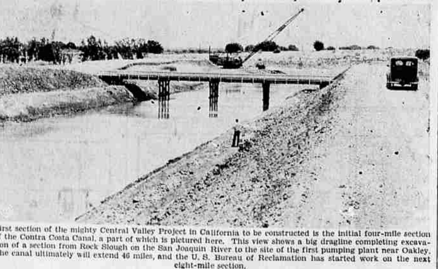
First section of the mighty Central Valley Project in California to be constructed is the initial four-mile section of the Contra Costa Canal, a part of which is pictured here. This view shows a big dragline excavating a section from Rock Slough on the San Joaquin River to the site of the first pumping plant near Oakley. The canal ultimately will extend 40 miles, and the U. S. Bureau of Reclamation has started work on the next eight-mile section.
