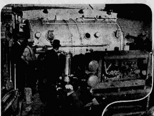
Divers going to the rescue of crews trapped in sunken submarines have been known to descend as deep as 300 feet below the surface. Above is pictured a recompression tank, in which divers suffering from the "bends" are given emergency treatment. At the right, Bill Reed prepares for one of his perilous descents. Below, the fleet submarine rescue and salvage ship, U. S. S. Ortolan, sends down a diver. Although unarmed, the Ortolan is an indispensable unit of Uncle Sam's battle squadron at sea.
