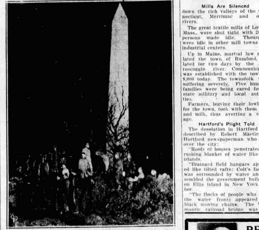
Dirt dikes and sand bag barricades were rushed up around all government buildings and property in Washington, D. C., in effort to forestall flood damage from rising waters of the Potomac river. These workers are shown in Potomac Park with the Washington monument in the background.
