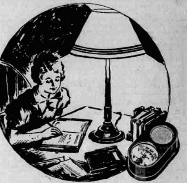
The Sight Meter, an instrument for measuring light, reads 20-30 footcandles under an I.E.S. Study lamp.
