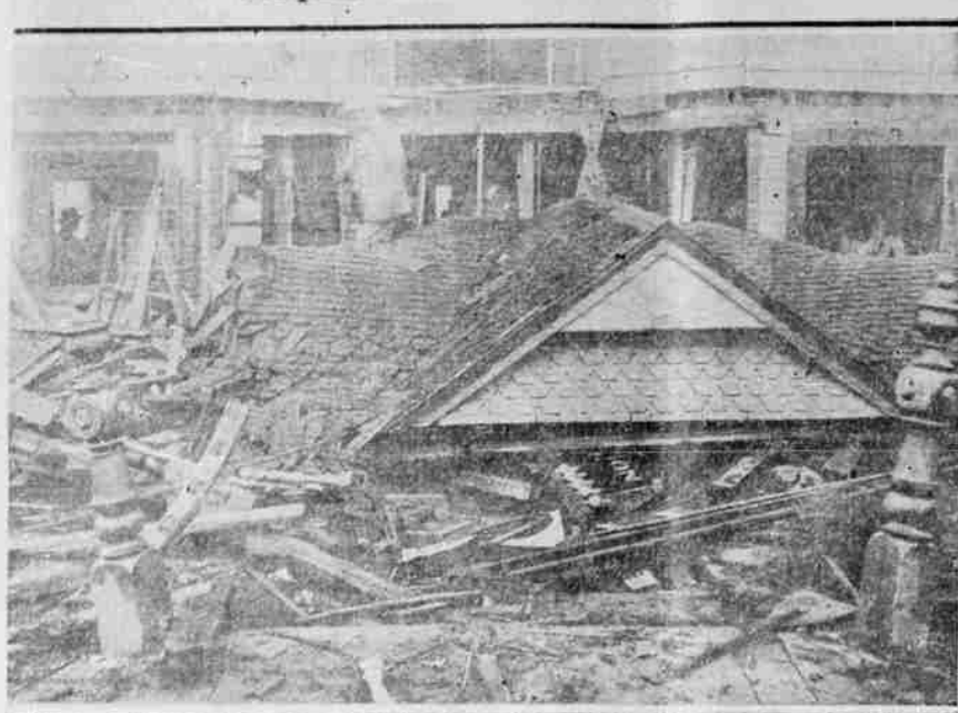
First and exclusive photo showing huge damage wrought by bomb which shattered the facade of the Filipino club at Stockton, California, Thursday night. Bombing marked a new outbreak of the anti-Filipino war in cities of northern California.
