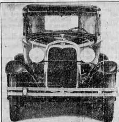
All exposed metal parts on the new Ford bodies are of rustless steel. Photo shows the new Tudor sedan.
