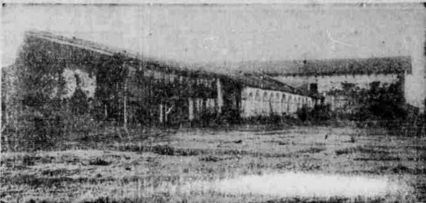
The famous San Miguel Archangel mission founded in 1731 is in imminent danger of collapsing. Termites, eating at unprotected wood, have brought the old structure to a critical point, according to C. James Lansing, secretary of the California Restoration society. An appeal is being made for funds to repair the building.
