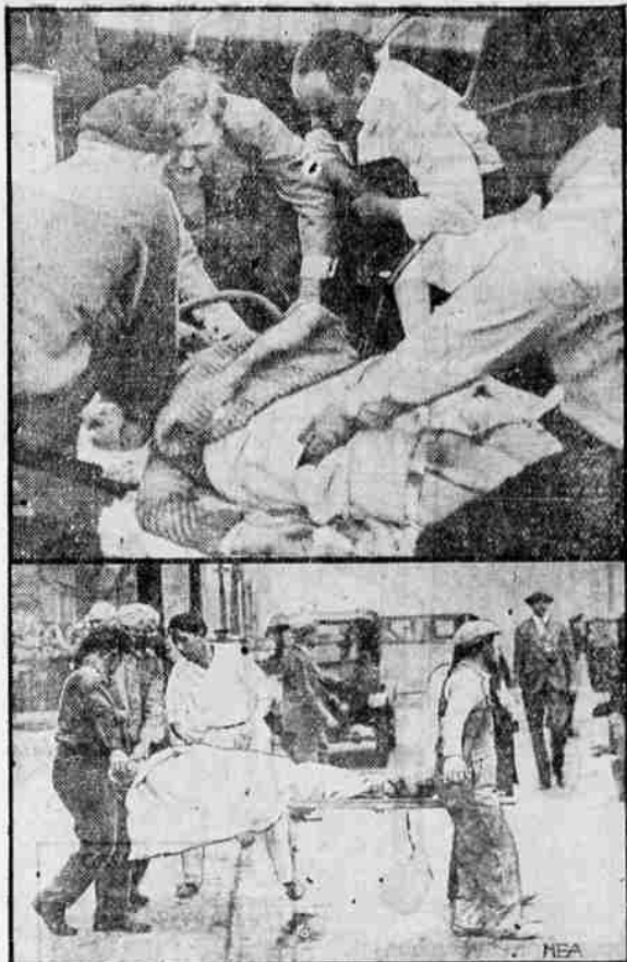
Doctors and firemen worked desperately trying to save the lives of victims of the explosion and fire that killed more than 120 people at Cleveland Clinic hospital. Victims are shown as they were stretched on the lawn in front of the building. In the center, volunteer stretcher bearers are carrying an injured patient to be taken to another hospital. Below, doctors and firemen are applying the pulmotor to one of the injured patients.
