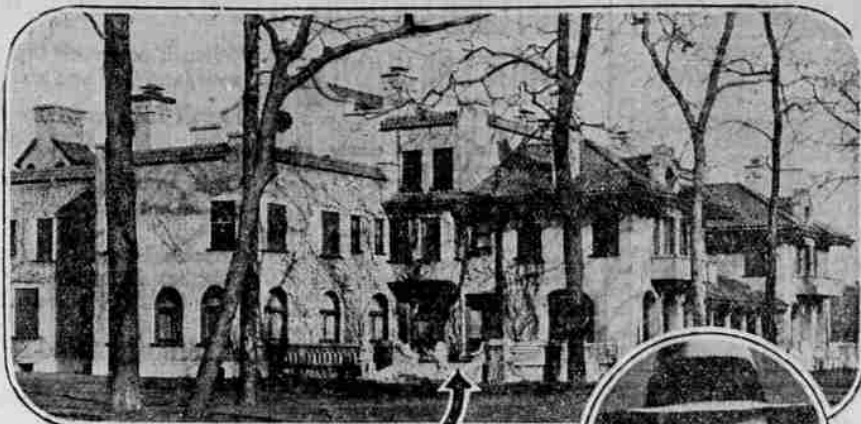
FROM THIS TO THIS
