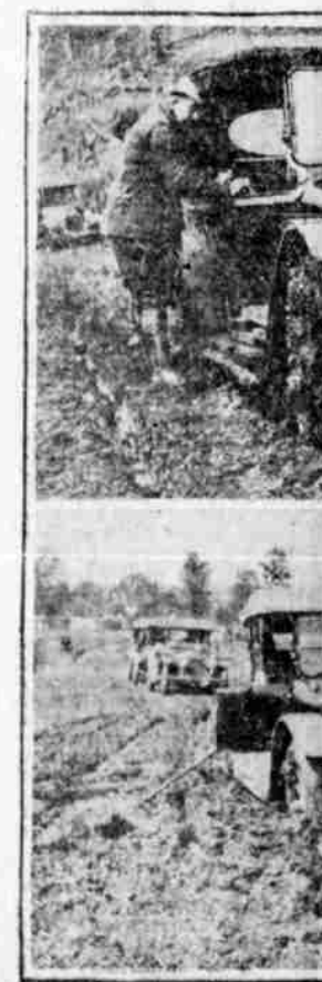
Above—Photograph of a Winson car taken in 1916 on the Pacific highway south of Roseburg-Glendale canyon below—Cadillac stuck in the mud at the same time and the same place.
