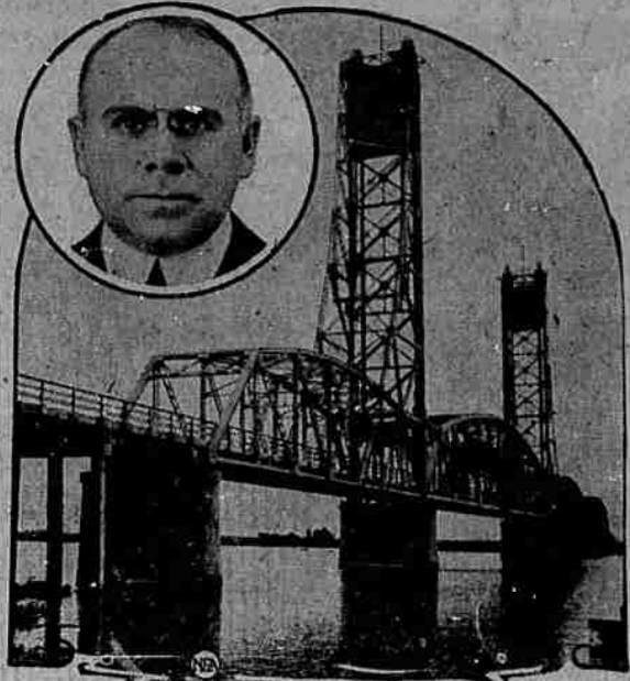
This is the kind of bridge that Thomas H. MacDonald, shown in inset, wants maintained over the streams crossed by federal aid roads. It's a toll bridge, but it will remain so only until its cost of construction is defrayed. It is the 10-mile Cochrane bridge over Mobile Bay.
