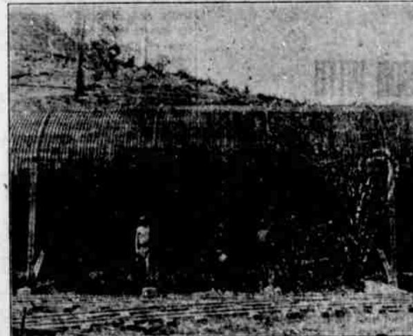
Wood Stave Pipe line Copco Two Plant, This 16-foot pipe is the largest on earth.
