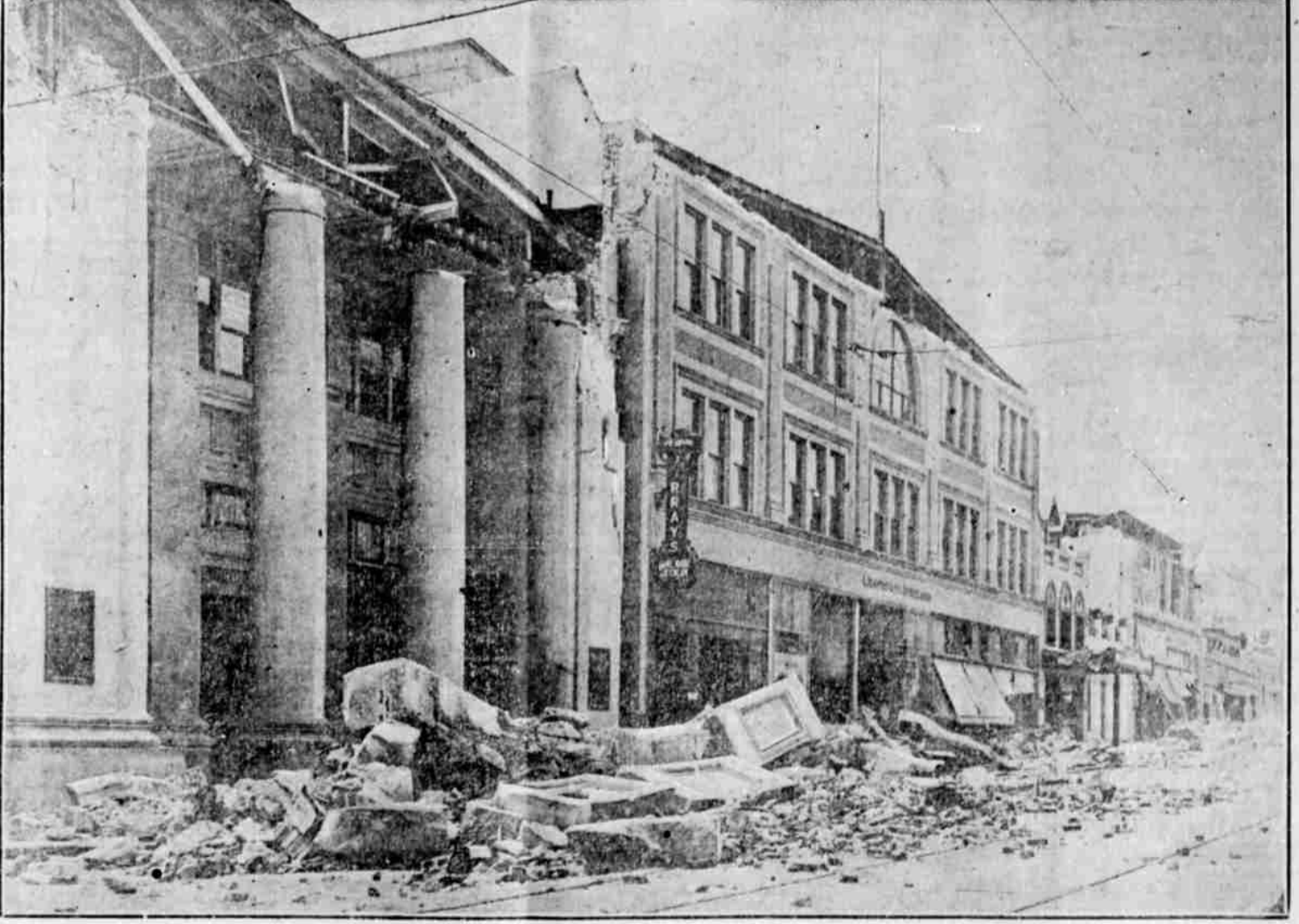
WRECKAGE—NOTHING BUT WRECKAGE—THE PHOTO SHOWS THE FRONT OF THE FIRST NATIONAL BANK BUILDING ON STATE STREET, SANTA BARBARA. THE CAVED-IN ROOF AND STATLEY COLUMNS BADLY DAMAGED ARE SHOWN. TODAY'S QUAKE SHOOK THESE COLUMNS AND WRECKED ONE OF THEM COMPLETELY. THE BUILDING WILL HAVE TO BE RAZED.
