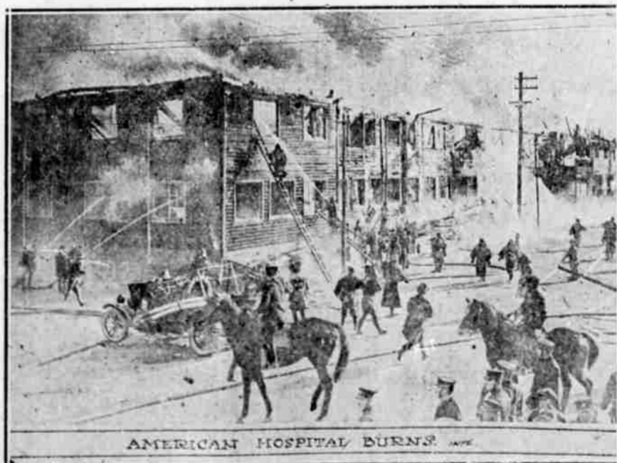
Above is shown the fire that destroyed St. Luke's Hospital, operated by the American Episcopal Church Mission, in Tokio, Japan. The building, a temporary structure used since the earthquake and fire of 1923, was gutted with a loss of $150,000. This remarkable photo was taken just as the roof crashed in with a roar.
