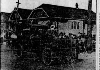
leials of the Chicago elevated railway lines have tested a new safety for railroad crossings which is said to be "fool-proof" against the careless le driver who now and then drives through the old-fashioned wooden and wakes up with a harp. The new gate will not allow an automobile ass. If a car runs into it the gate gives several feet and then bounces car back like a rubber bull.
