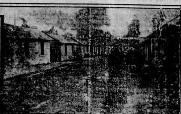
VIEW IN RESTORED SECTION OF PERONNE, RAZED BY GERMAN SHELLS
