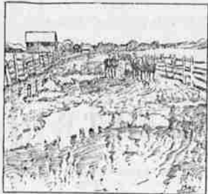
TYPICAL CLAY ROAD BEFORE IMPROVEMENT.
