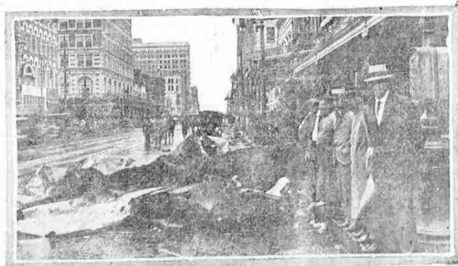
MAIN ST., HOUSTON, TEXAS, SHOWING DEBRIS FROM ROOFS AND BUILDINGS PILED IN STREET. A $1,000,000 PROPERTY LOSS HAS BEEN REPORTED FROM HOUSTON.
