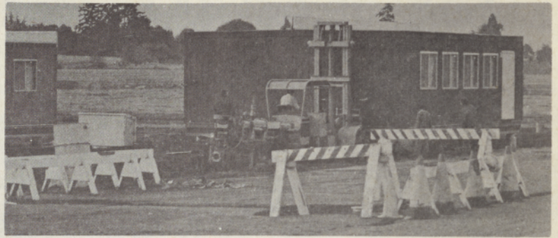
Six temporary classrooms have been erected East of Chugach Street.
