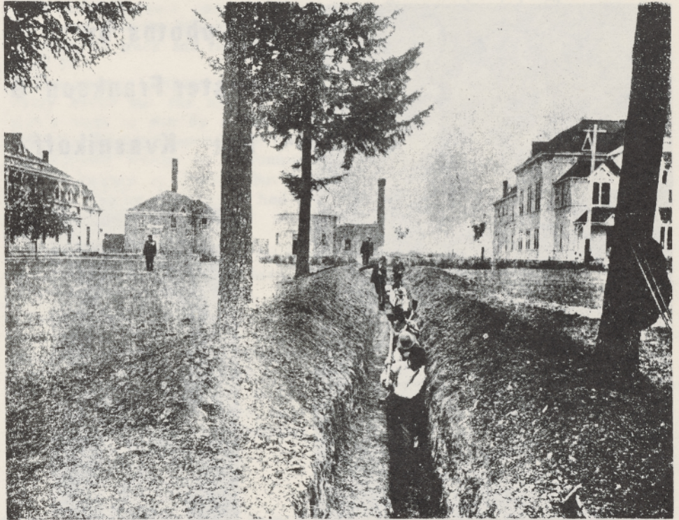
Back when a lot of today's troubles began--Turn-of-the-century Chemawa students lay some of the original pipes the hard way, with picks, shovels and a lot of muscle. Today one backhoe does the job faster. (Photo courtesy Chemawa Archives)
