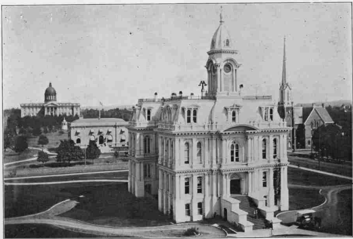
MARION COUNTY COURT HOUSE. SALEM, OREGON.
