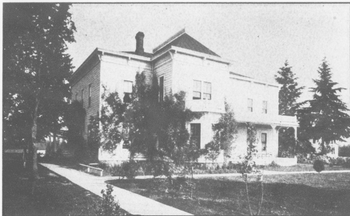
EMPLOYEES' BUILDING, CHEMAWA.
