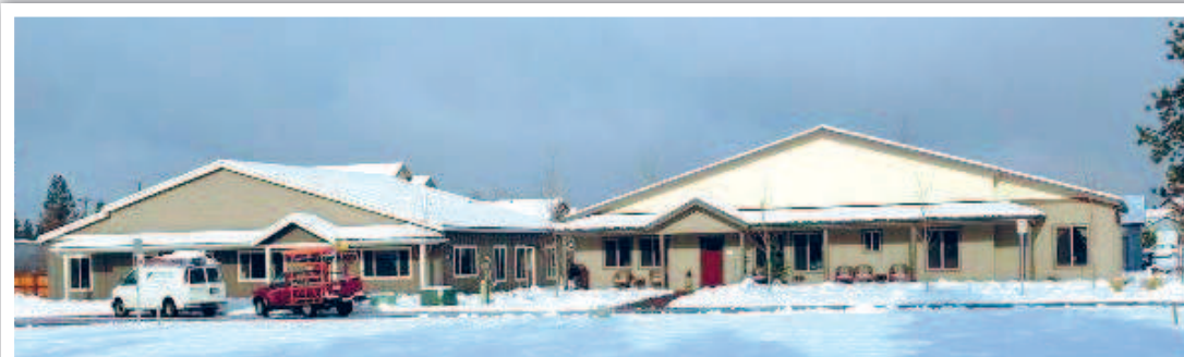
Final detail being completed on Pennington’s Place
