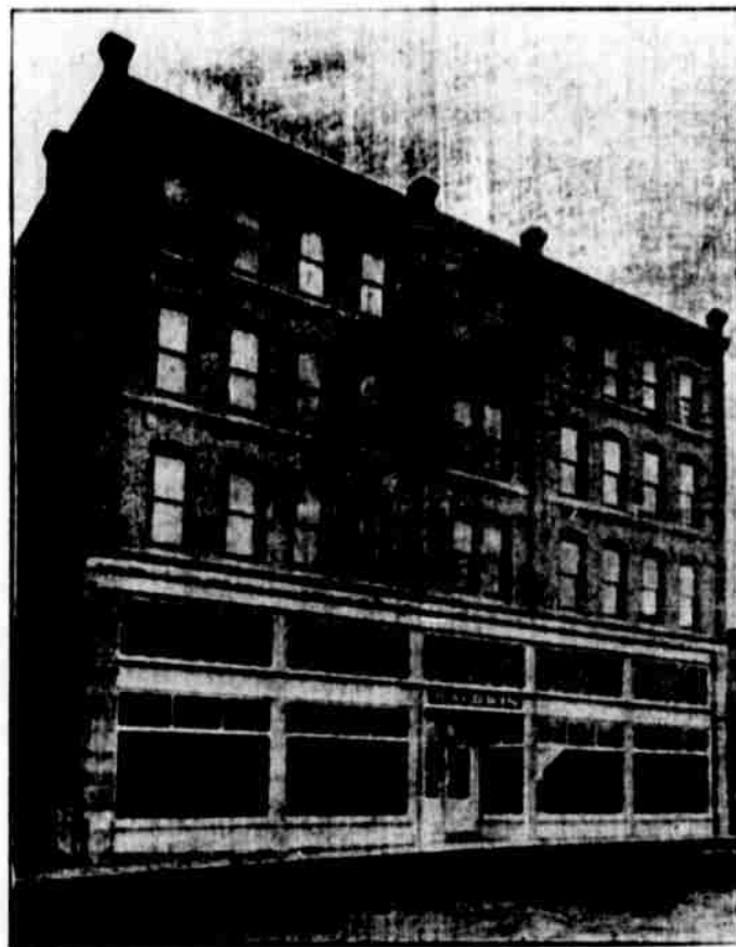
BALDWIN BLOCK, WHICH MAY BE CONVERTED INTO A FINE MODERN HOTEL.
