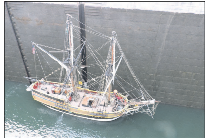
The Lady Washington sits at the bottom of the McNary Dam locks while passing through the dam on Monday.
