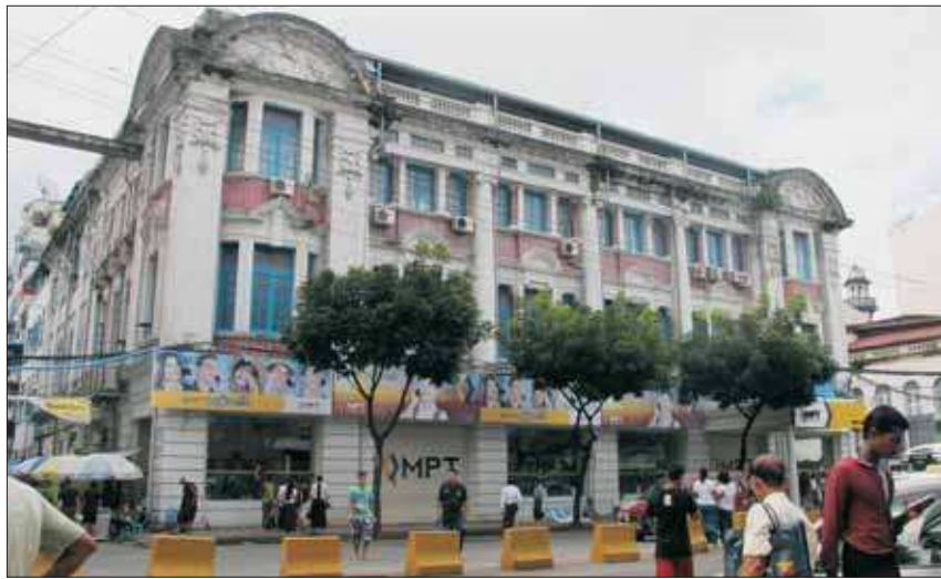
LAST BEST CHANCE. People walk by an old colonial building used by Myanmar Posts and Telecommunications (MPT) as an office in Yangon, Myanmar. The Yangon Heritage Trust says Myanmar's largest city and commercial capital is facing its "last best chance" to salvage and restore many crumbling colonial treasures. It has proposed a heritage strategy for the city that outlines a vision of how to make the city more livable, modern, and affordable, while preserving its unique landmarks and neglected green spaces. (AP Photo/Elaine Kurtenbach)
