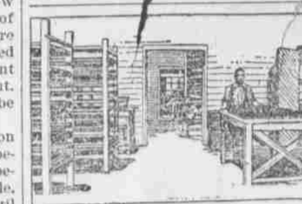
ROLLING AND DRYING ROOM.
