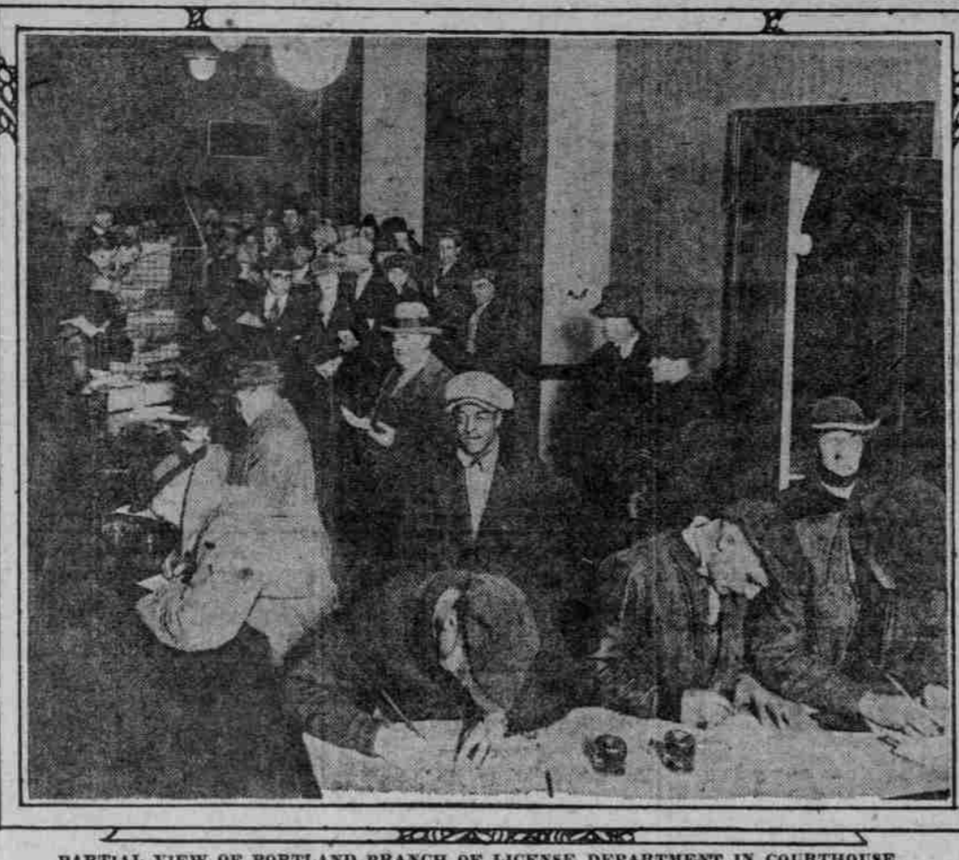
PARTIAL VIEW OF PORTLAND BRANCH OF LICENSE DEPARTMENT IN COURTHOUSE.
